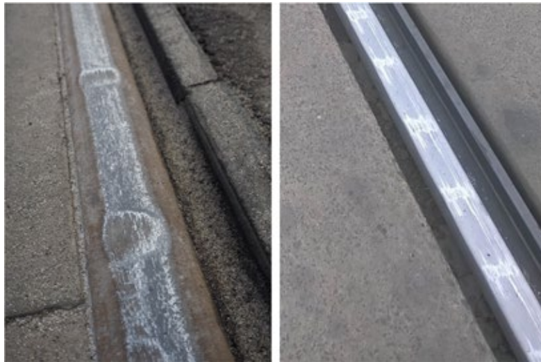
Fig. 1. Common rail defects of grooved rails
