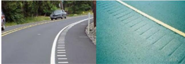
**Fig.2.** Raised (Left) and Rolled-in (right) Rumble Strips
