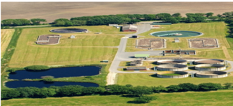
Fig. 2. Facility for Waste Water Treatment in Kukshaven, Germany Source: Modified from (Waste water, 2017)
