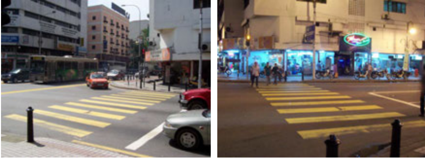
Fig. 2. Signalised Crosswalk that is Located along Jalan Putra (Putra Road) during Daytime (L) and Night Time (R)
